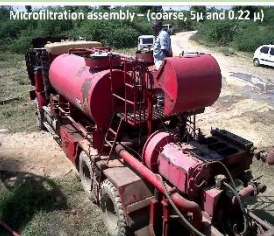
Microfiltration assembly – (coarse, 5µ and 0.22 µ)
